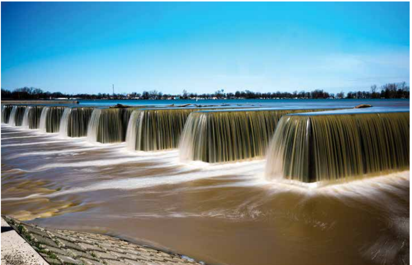
Labyrinth spillway at Indian Lake State Park.
