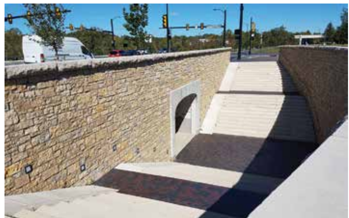
In Dublin, Ohio, this aesthetically enhanced pedestrian underpass tunnel below Riverside Drive provides a safe connection between the new parks and the Bridge Street District.
