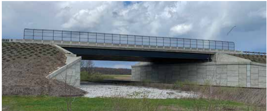
EMH&T designed a 149-foot single span plate girder bridge over CSX railroad tracks, which facilitated semi-integral abutments behind MSE walls, architectural enhancements to the bridge railing, and pedestrian facilities on both sides of the roadway. EMH&T's rail engineers also provided coordination with CSX throughout the project.
