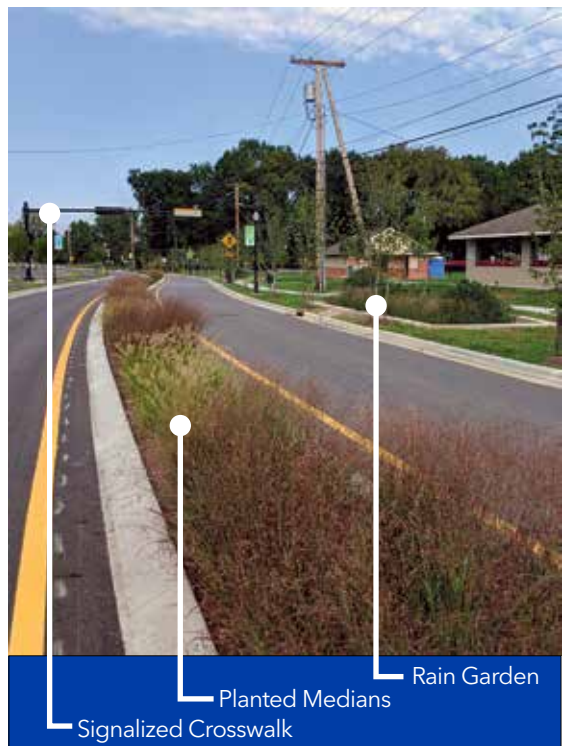
Road reconstruction projects present opportunities for placemaking, as well as safety installations and green infrastructure elements.
