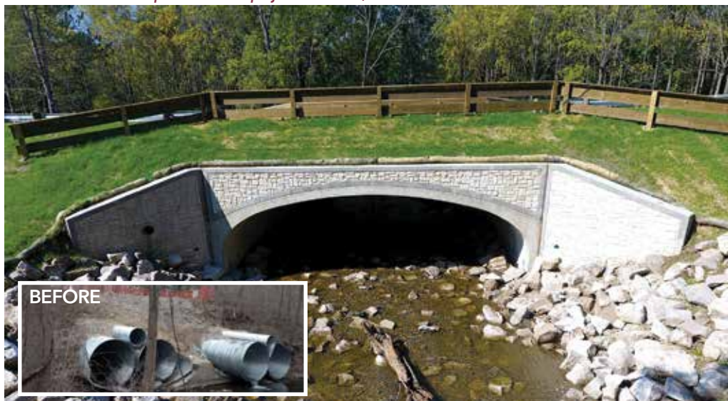
Guilford Road culvert replacement LPA project in Medina, Ohio.
