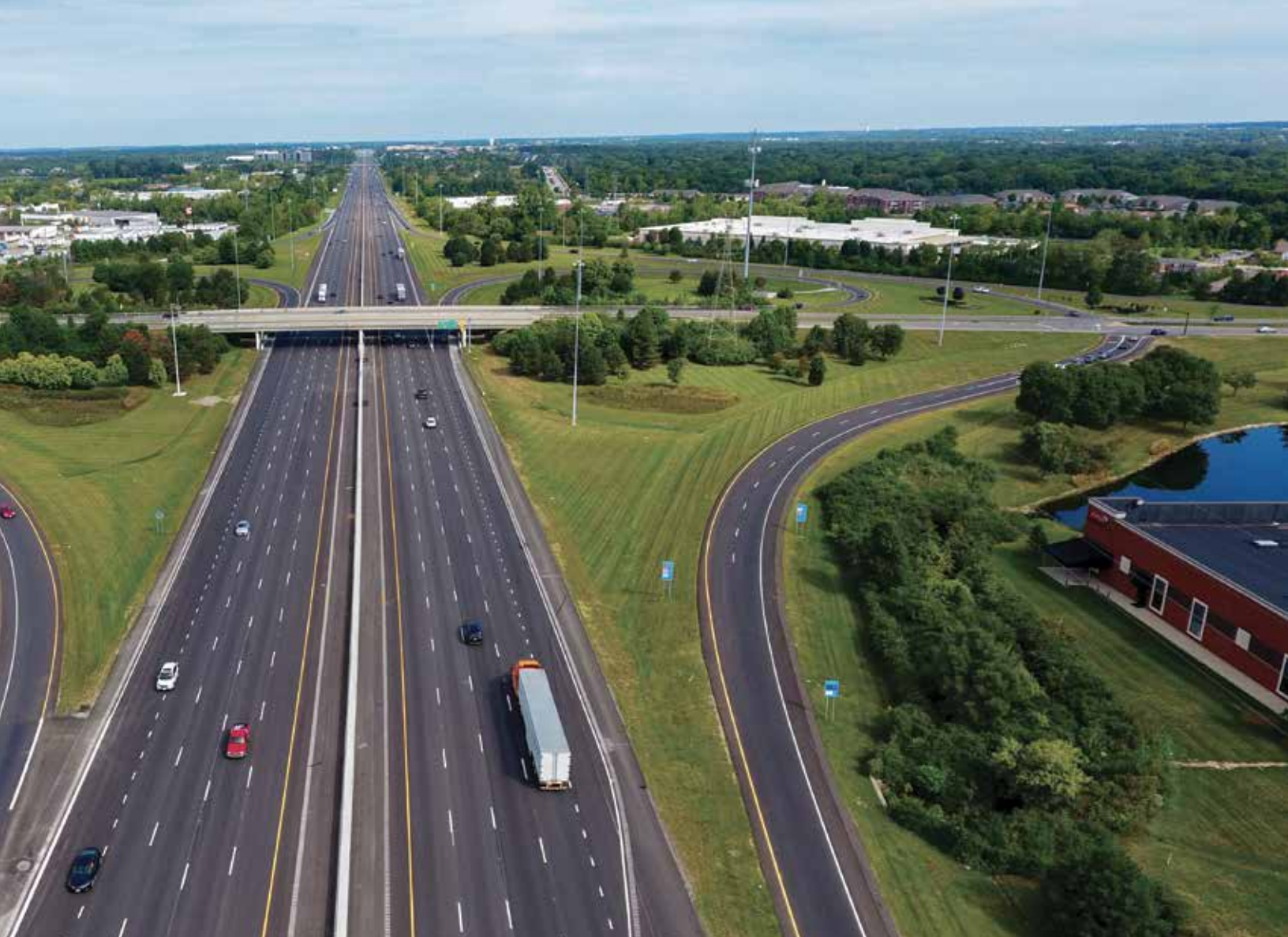
EMH&T provided a design solution for the I-270 Northwest Side Widening project in Columbus, Ohio, which included closing the median with barrier on this 8-mile stretch of highway and adding an additional lane in each direction.
