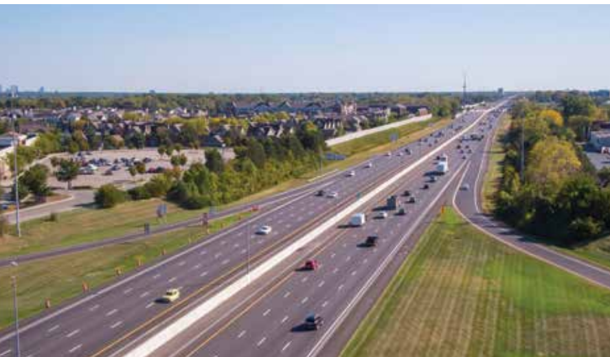
The project included the widening of three mainline bridges, full depth pavement repairs, noise wall design, continuous highway lighting, and upgraded signage and Intelligent Transportation System (ITS) facilities along the corridor.
