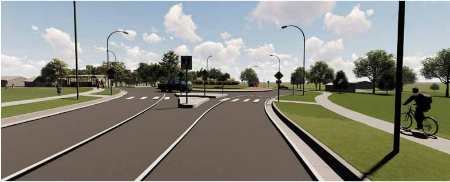
This approach view of a new roundabout in Strongsville, Ohio, allowed engineers to visualize the line of site at the facility approach.
