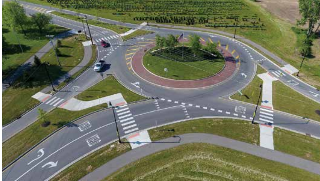
Gender and Lithopolis Road roundabout LPA project in Canal Winchester, Ohio.
